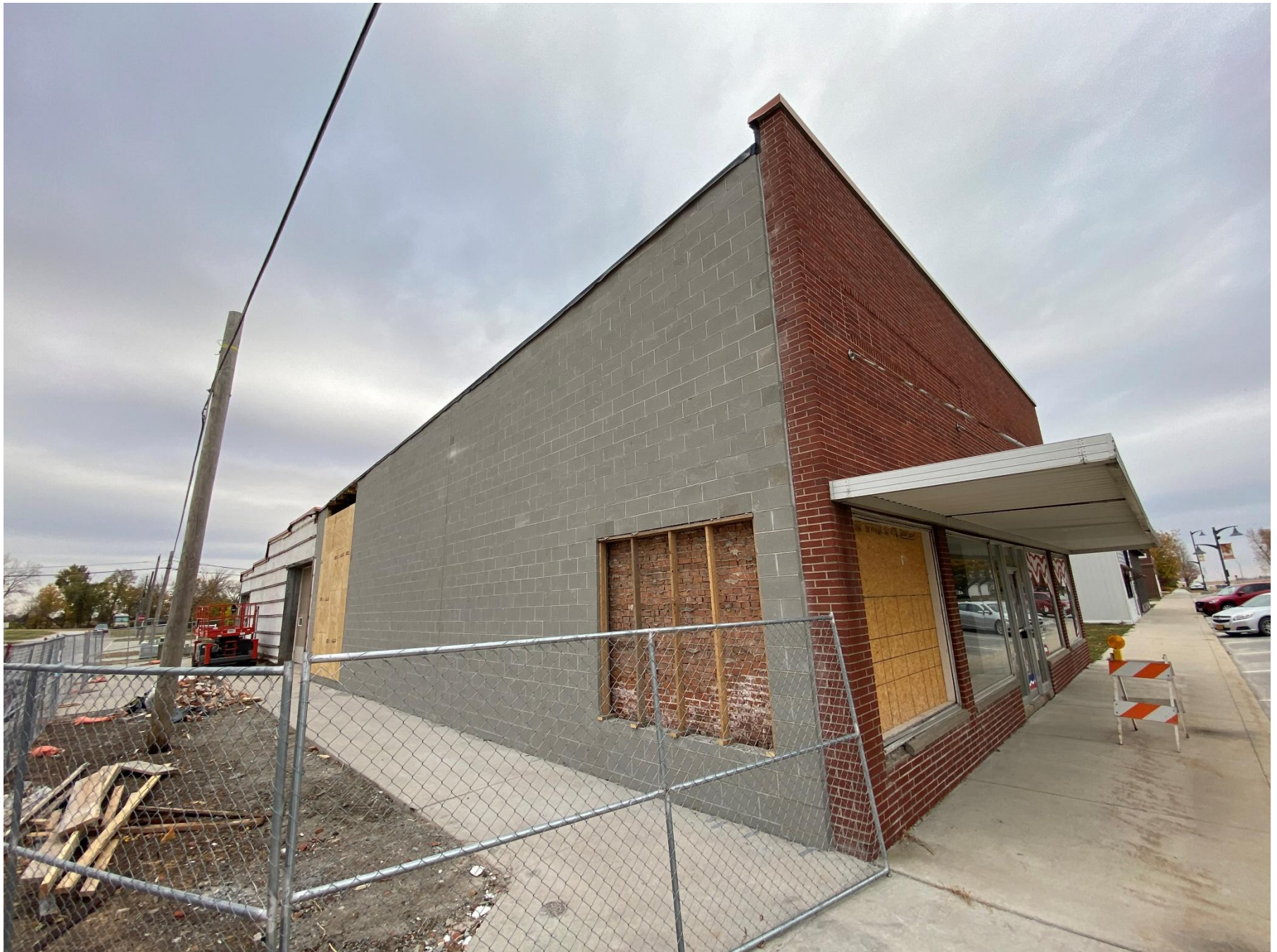
(West Wall Restoration – Fall/2024)
