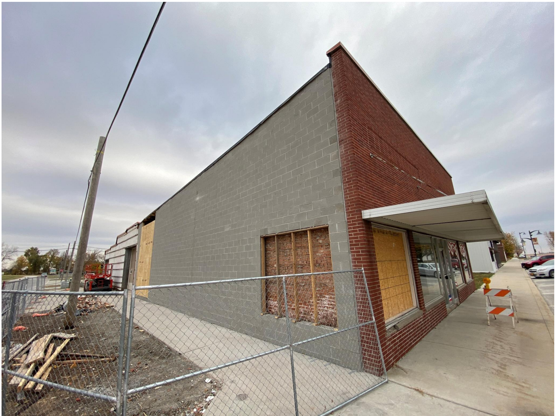
(West Wall Restoration – Fall/2024)
